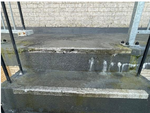
The damaged sections of concrete will need to be repaired.
