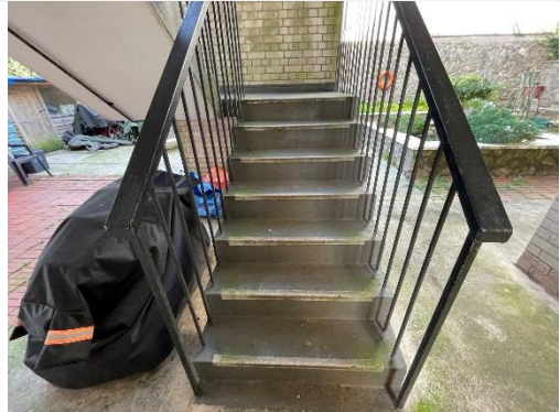
Overview of the staircase. The edge of the stairs shall be coated in yellow.
