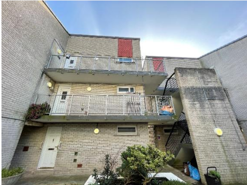
Overview of the balcony area. The system is no longer providing adequate protection.
